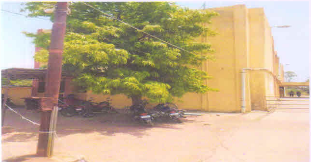
Pic -7 Side Area
